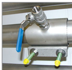
B Spot drilling collars
